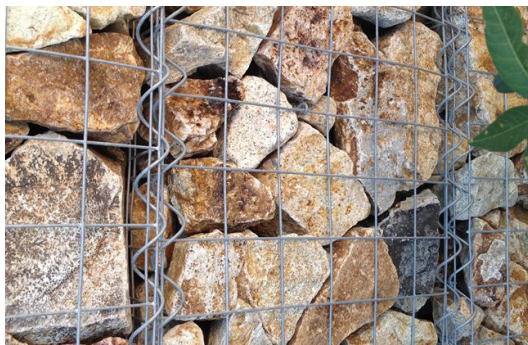
Custom mix gabion retaining wall (re-use onsite materials)
