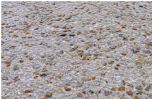
Insitu concrete with custom aggregate mix
