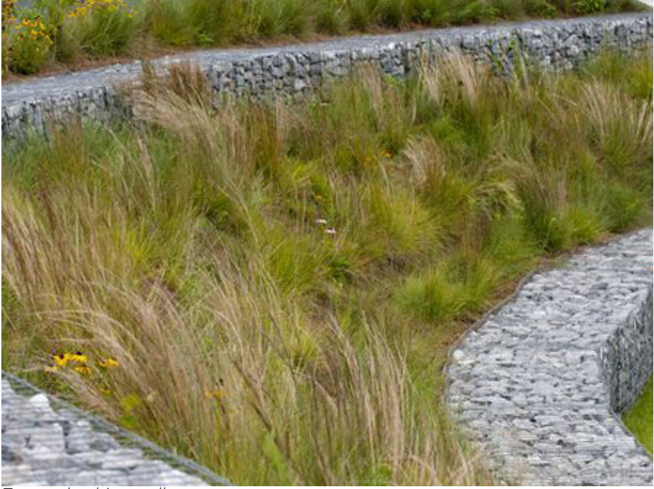
Terraced gabion walls
