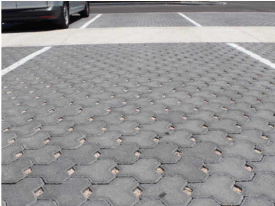
Permeable paving to drop off zone
